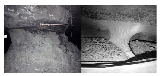
**Figure 5.** Views of damaged mine workings with inclined sidewall surfaces: (**left**)—long pillar at an intersection in Rudna mine, (**right**)—sidewall of a rectangular gallery with inclusion of competent rocks—Polkowice-Sieroszowice mine after blasting works in the close neighborhood, February 2016.
